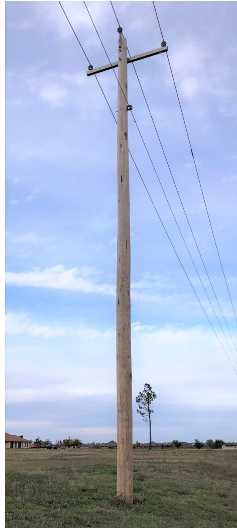
Proposed Distribution Structure
